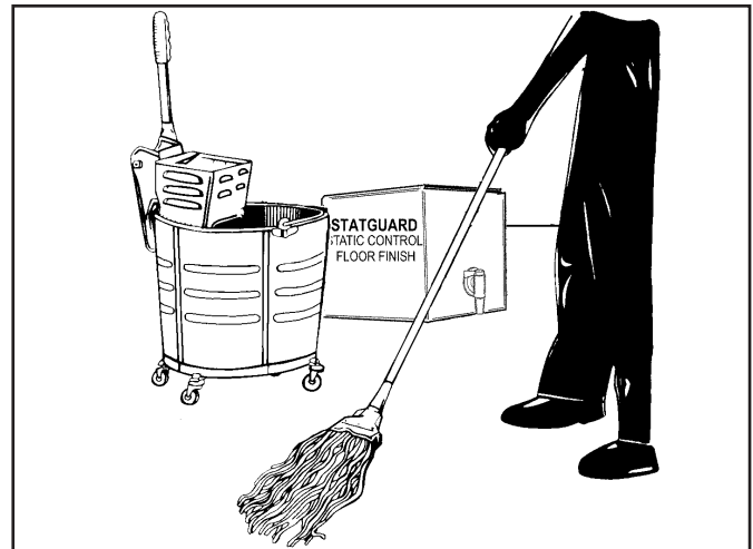
Figure 4. Applying floor finish.
